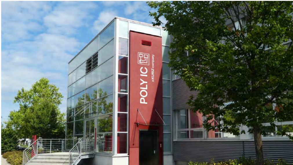
Ill. 30: POLY IC company premises; source: KURZ
