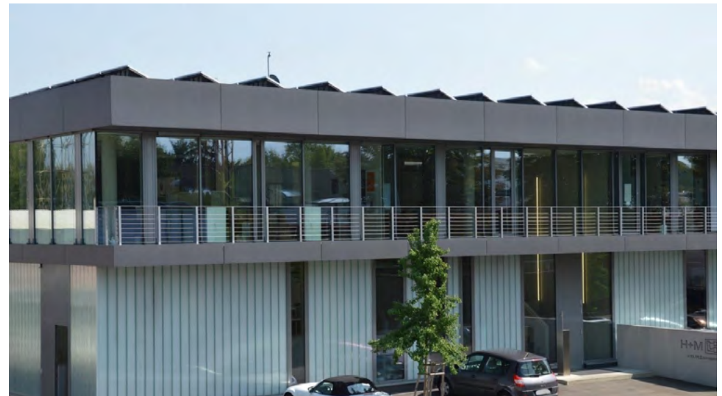
Ill. 20: H+M company premises; source: KURZ
