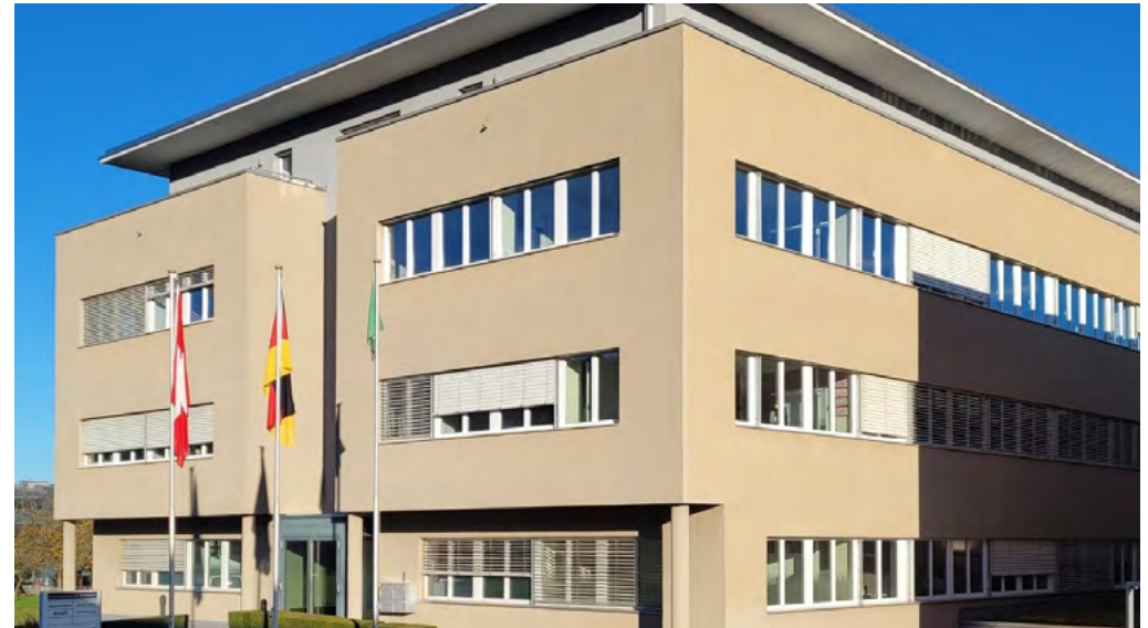
Ill. 36: STEINEMANN DPE company premises; source: KURZ
