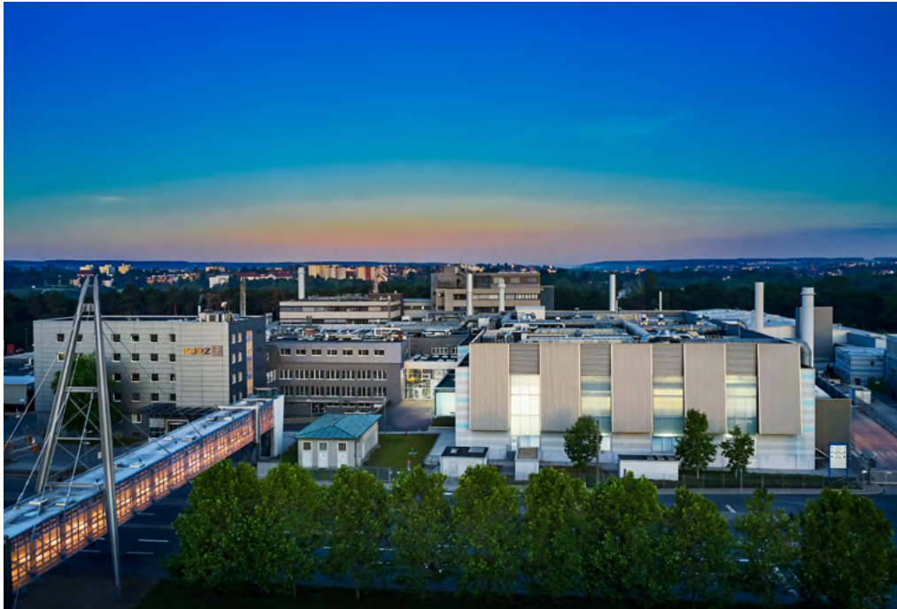
III. 11: Company premises in Fürth; source: KURZ
