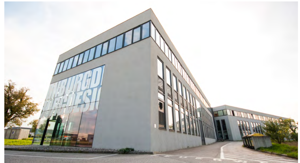
Ill. 16: BURG DESIGN company premises; source: KURZ
